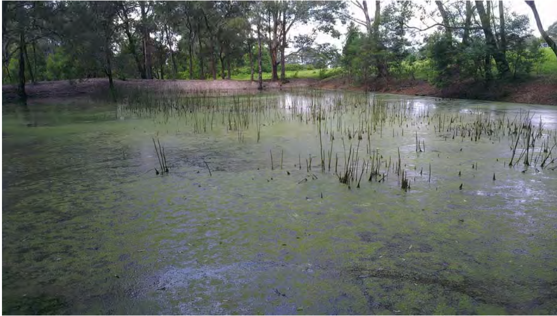
Photo 6 – The dam looking south east
